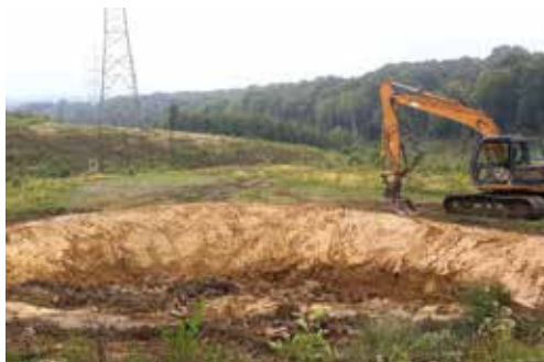
Pond dug in the best way to favour biodiversity: orientated to the south, with mild slopes along the banks and in a bean-shape
